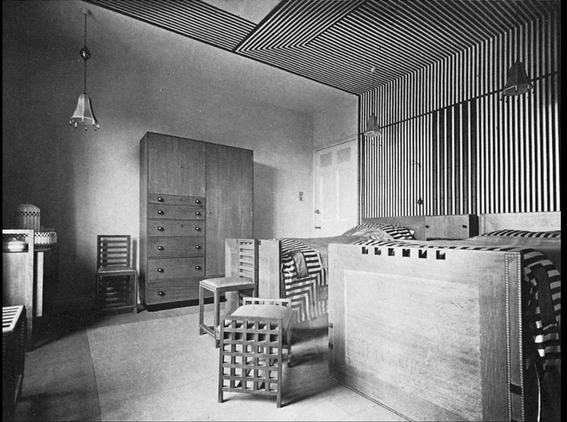
Charles Rennie Mackintosh – Casa in 78, Derngate – Northampton – 1916-17
